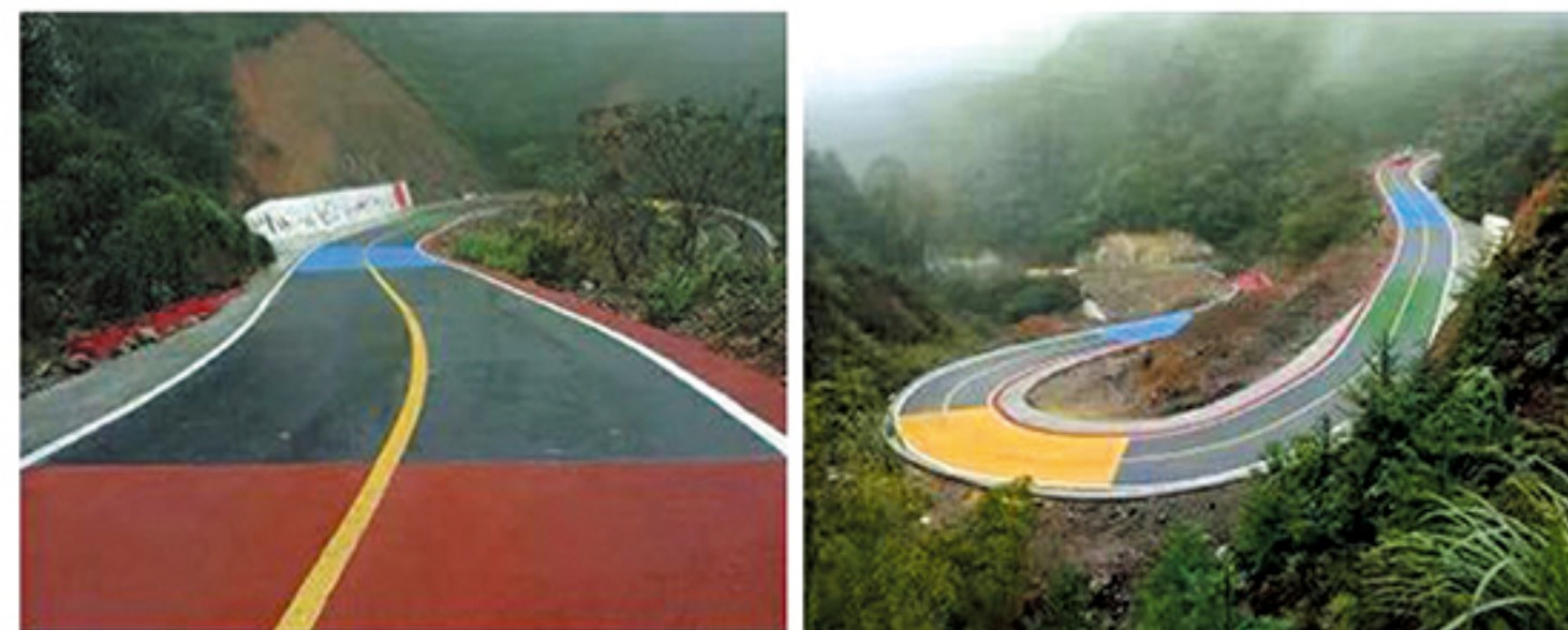
双组份彩色防滑路面标线 Double component color antiskid pavement marking
